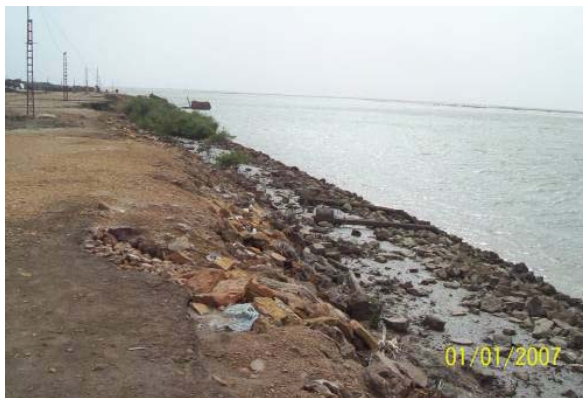
Proposed site for installation of tide gauge - New Jetty Construction site
