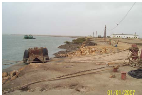
Ketti Bandar-Site inspection mission for tide gauge installation
