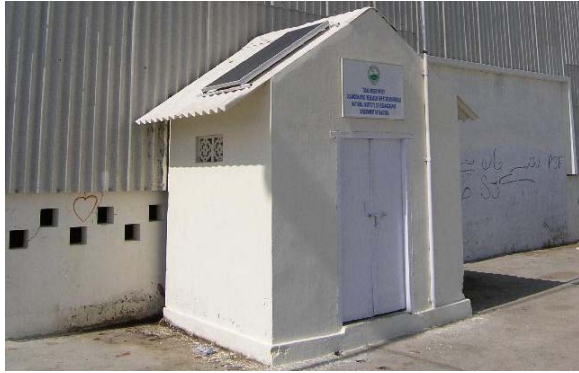
NIO-Tide Gauge installed at Gwadar Port
