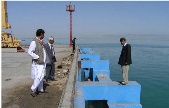
East End of New Gwadar Port-Site inspection visit for Tide Gauge installation
