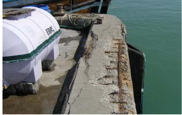
South West End of Fish Jetty at Gwadar port
