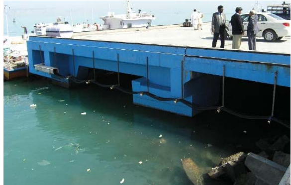
West End of New Gwadar Port-Site inspection visit for Tide Gauge installation
