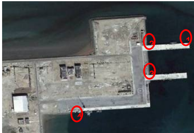
Figure 2: Ormara Navy Port (from Google)
