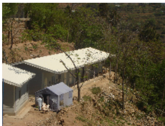
Photo 2: ICT, Library and Science Lab at GBHS Noorpur Nakran
