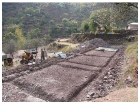
Construction of Government Girls High School Sharian
