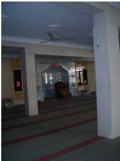
Mosque (note reinforcing pillars)
