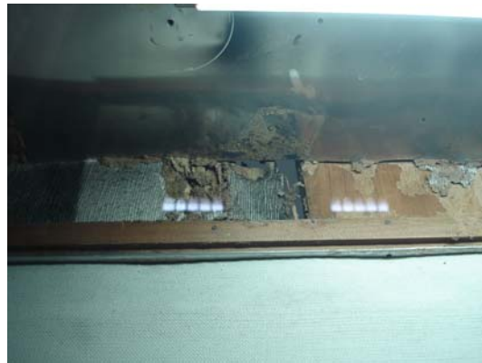
Fig. 1.10- Termite attack is seen in some of the display cabinets.
