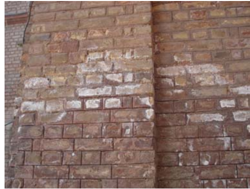
Fig. 1.2 - Efflorescence seen at the rear of the building
