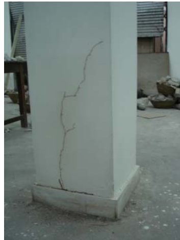
Fig. 2.4- Termite attack is observed in the storage
